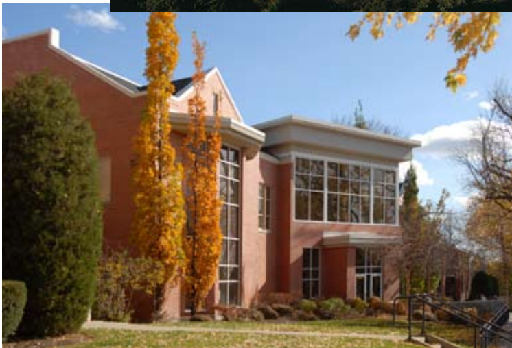
Building 114, of the Behavioral Health complex.
