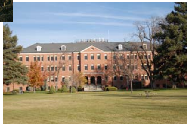
Building 67 of the VA Medical Center
